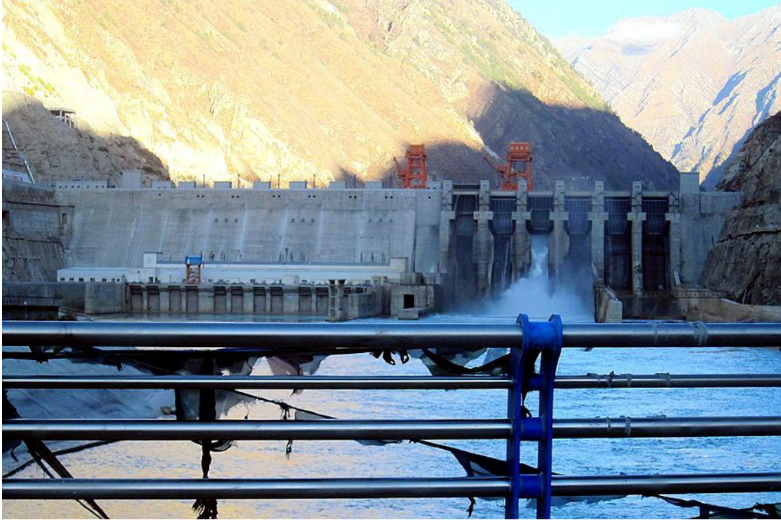
Completed dam (1) between Gyaca and Sangri 12/11/2016
