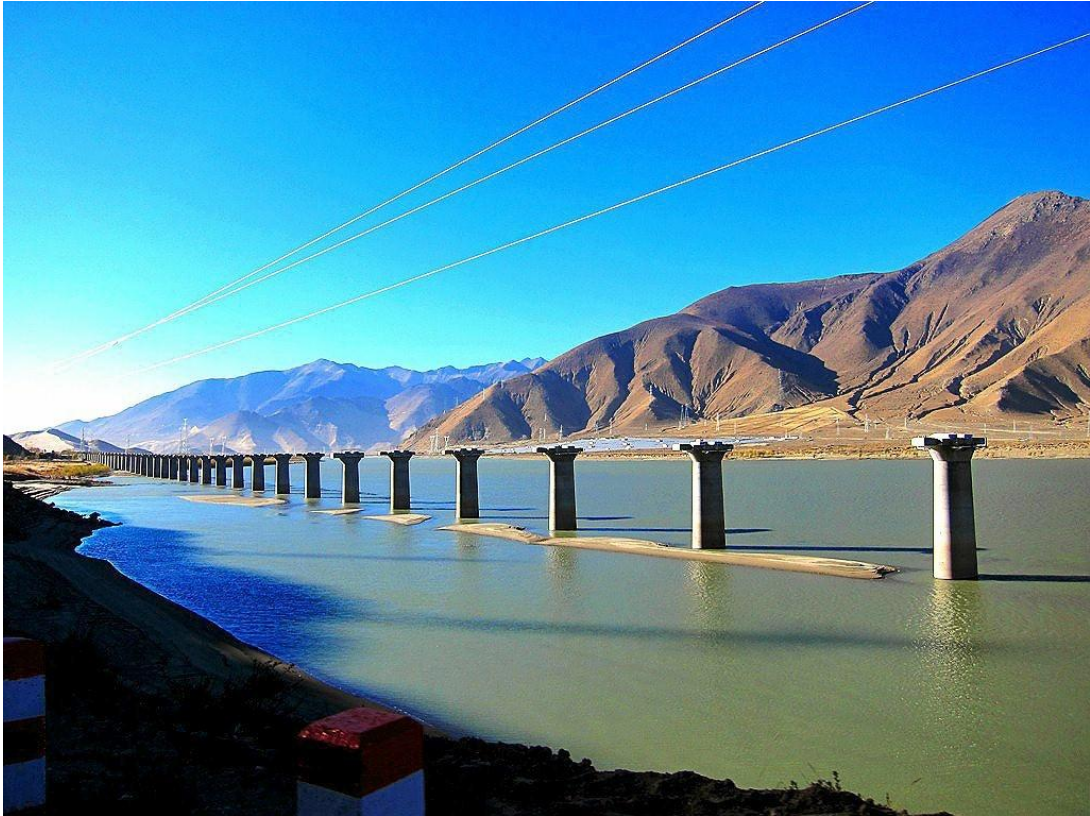
Railway construction on river stream between Sangri and Zetang 12/11/2016
