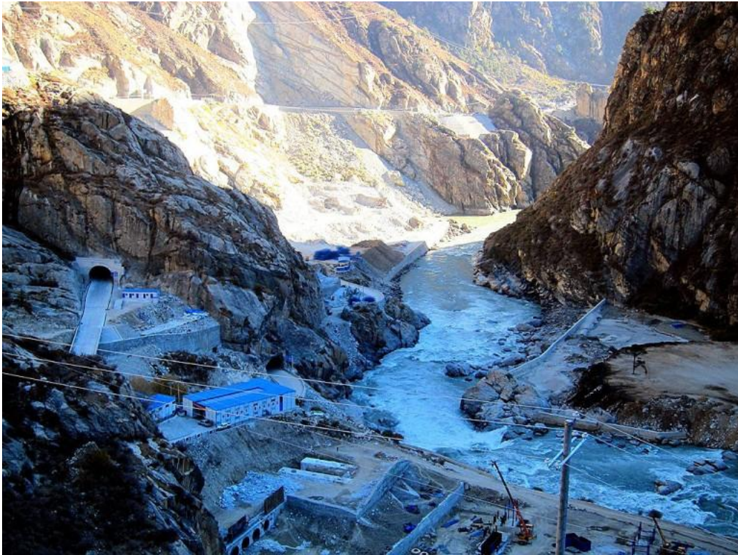
Construction site for new dam between Gyaca and Sangri 12/11/2016
