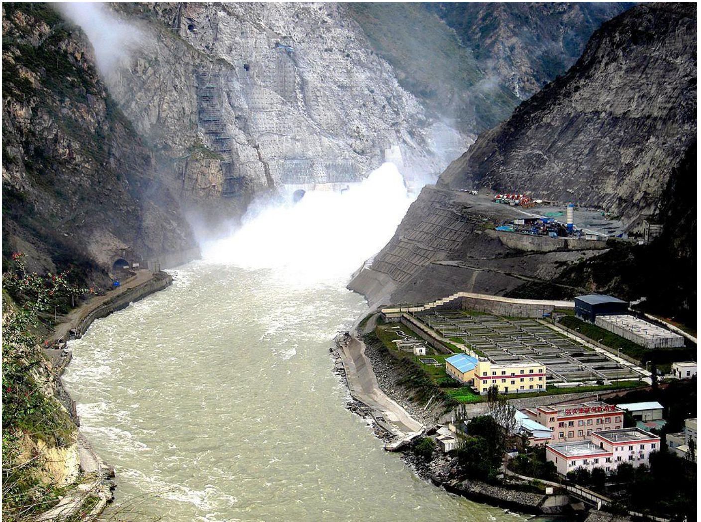
Base for dam construction, Dadu river, north of Luding, Sichuan
