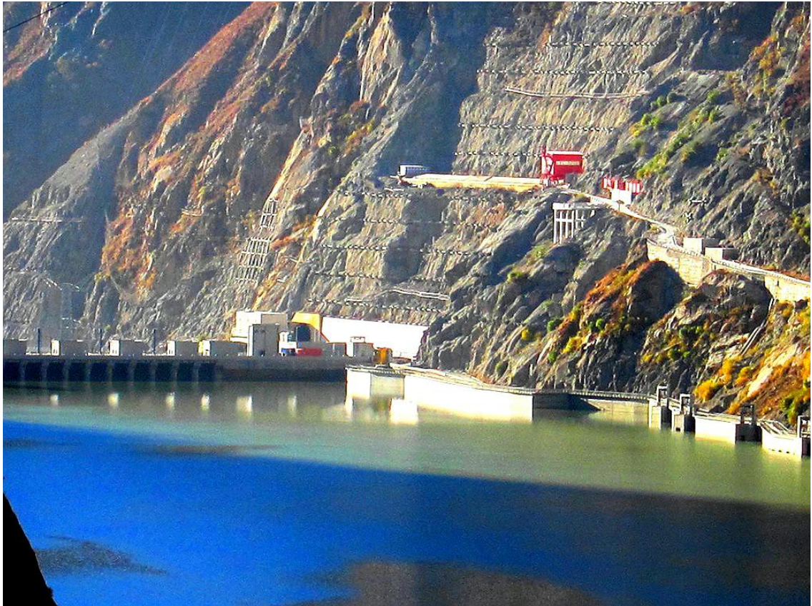
New dam constructed in Yarlung Zangbo west of Milin
