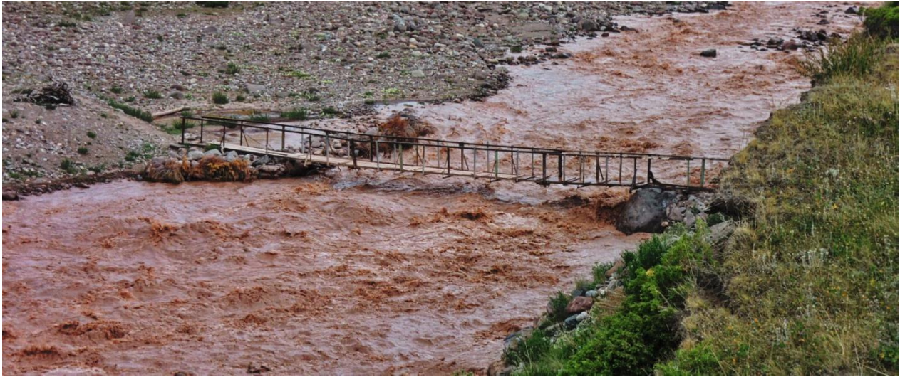
Pic. 13-33. Bridge across Nura River.
